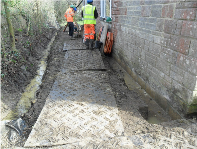
View of western boundary showing hedge trimmed back and ditch cleared.
