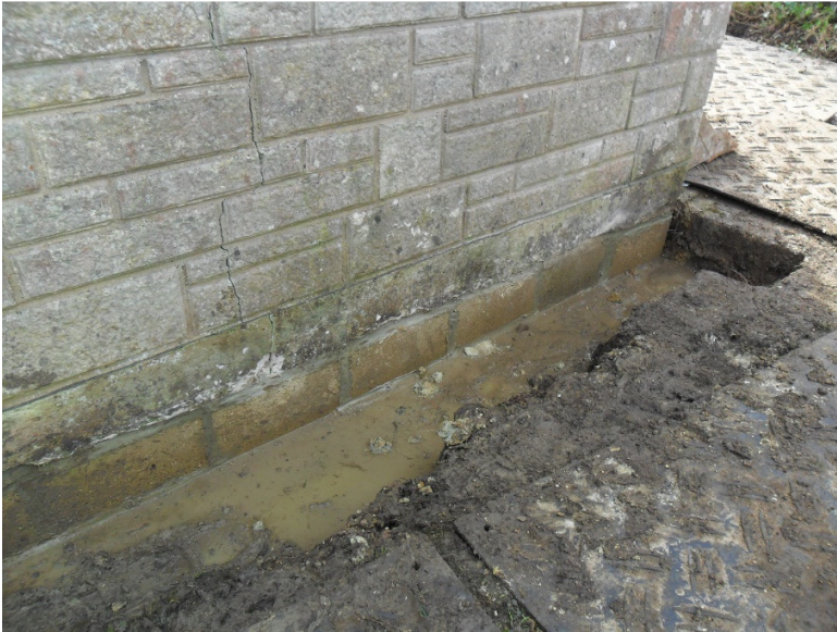
View of blocks replaced at base of wall.
