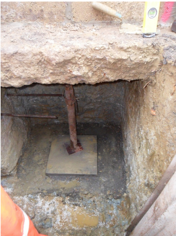
View of underpin excavation.
